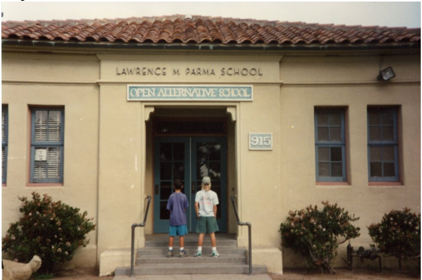
The now-shuttered Lawrence M. Parma School, Santa Barbara. Undated photo courtesy of Dennis M. Koski.
